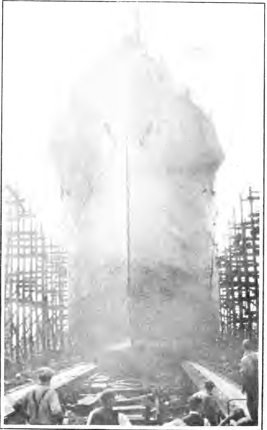
Launching of the S.S. "Munsmar." The picture was taken at the Moment the Steel Hull Started down the Ways.
